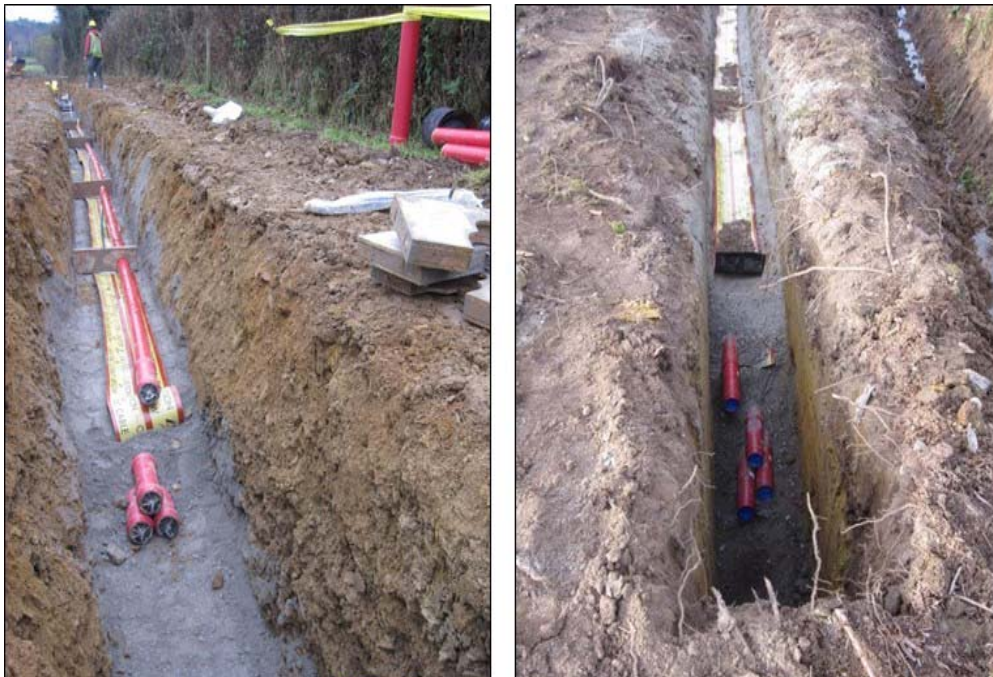
Plate 2.1 Cable Trench View
